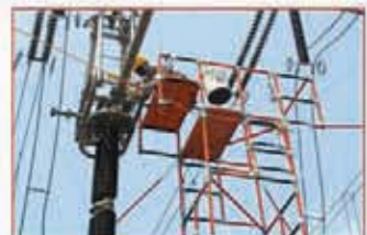
Maintenance of Pantograph Isolator in 400 kV Switchyard at Bhopal
