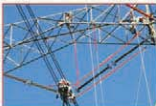
765 kV Quadruple Conductor-Insulator Change out at Mega
