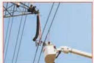
400 kV Suspension Insulator String Change out at Bhopal
