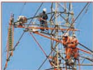
161 kV Suspension String Work using Trolley Pole in Ghana
