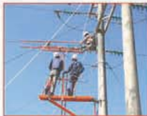
Use of Platform on 66 kV Tension Pole in Myanmar
