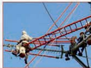
132 kV Tension Insulator String Replacement in Sri Lanka
