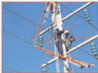
Application of Hot Stick Method on 66 kV Pole in Myanmar
