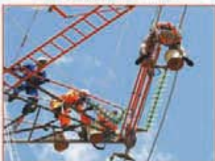
Use of Bare Hand Technique on 161 kV Tension Tower in Ghana
