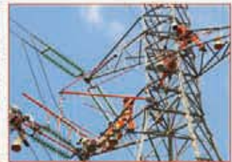
Use of Insulated Boom on 161 kV Line in Ghana
