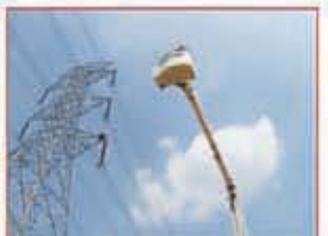
Insulated Aerial Platform for 400 kV Line Work at Bhopal
